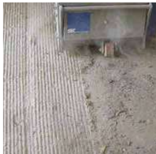
4 – Fresatura Milling
