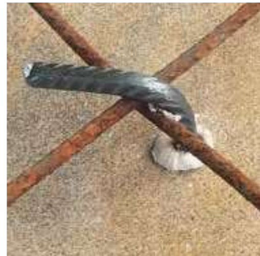
3 – Aggancio armatura + aggrappante Connection armor + adhesion material
